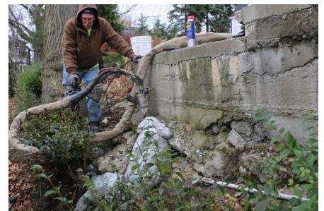
Injecting HydroFoam
