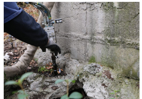
Injecting HydroFoam
